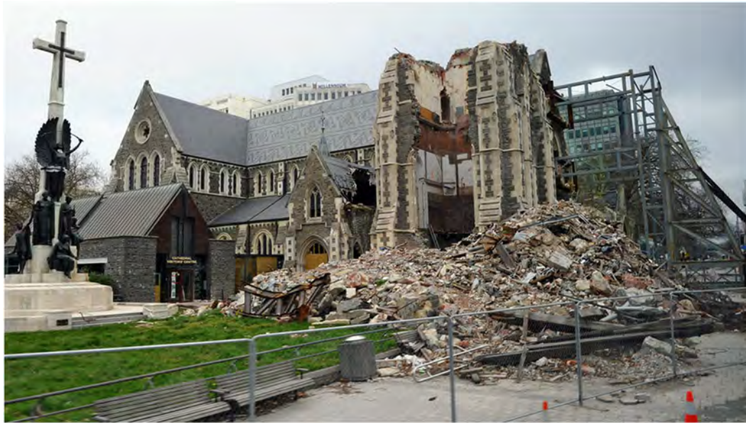
Fig. 114. Damage done to the cathedral in Canterbury, New Zealand, by the 2010 M 7.1 earthquake ( http://www.npr.org/sections/parallels/2015/04/05/397093510/will-new-zealand-rebuild-the-cathedral-my-forefather-erected ).
